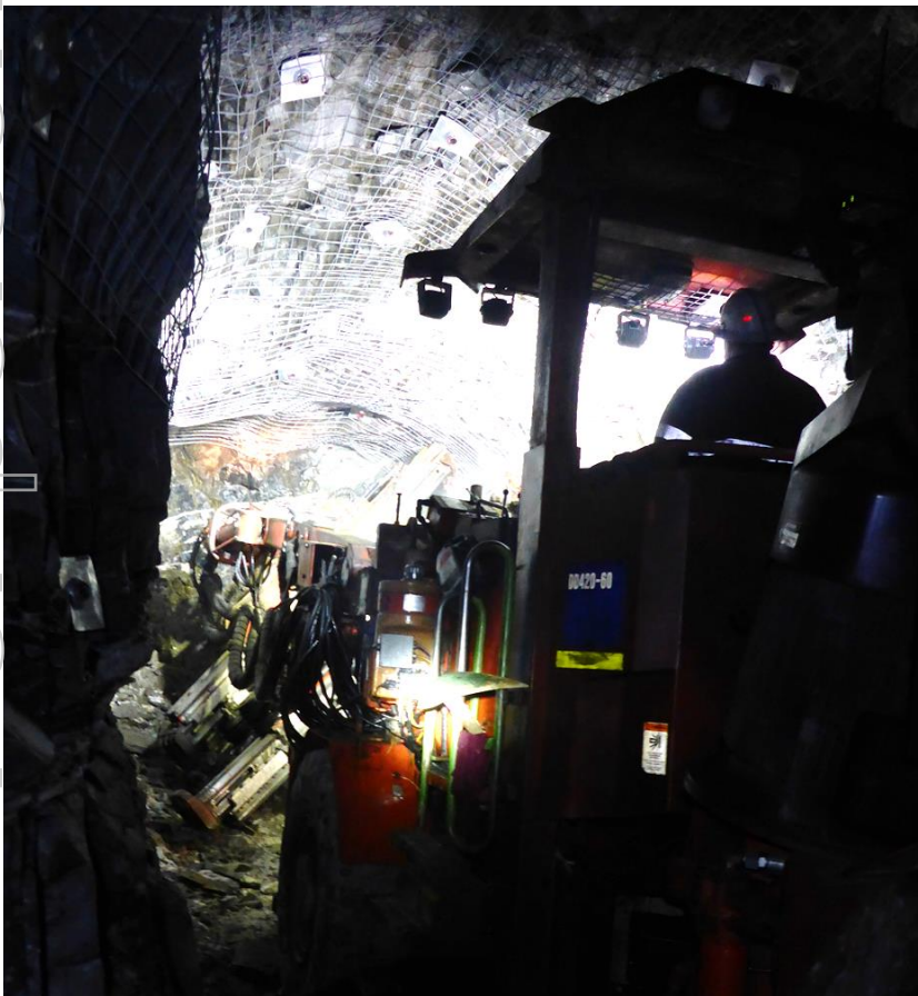
Figure 5. Mechanised (Jumbo) Development of the 1394 Ore Access Drive at the A1 Mine.
