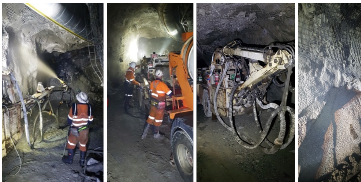
Figure 1: Images of Shotcrete application at A1 Gold Mine, June Quarter
