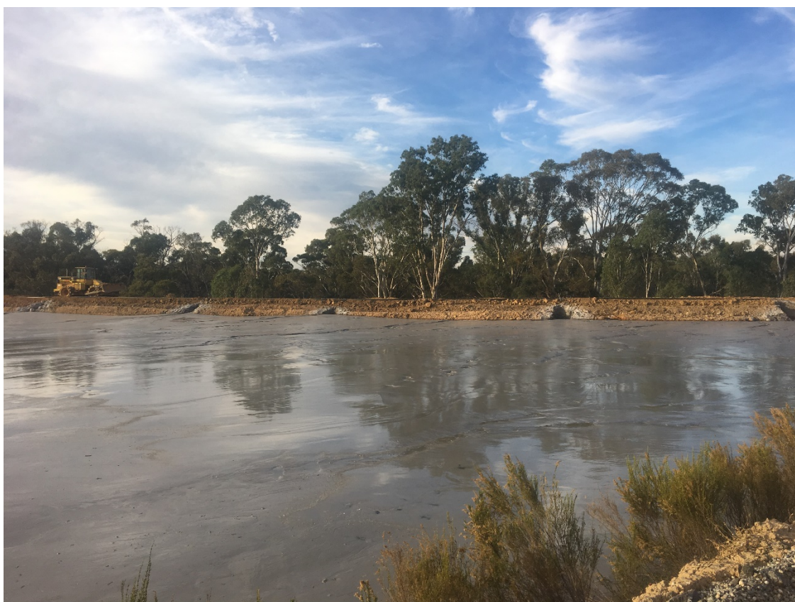
Figure 4: Southern Wall lift and tailings operation of TSF at Porcupine Flat
